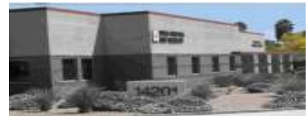
Hayden Business Center, 14201 N. Hayden Road Southeast Corner of Hayden and Scottsdale Roads
